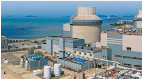
Ling-ao Nuclear Power Plant
